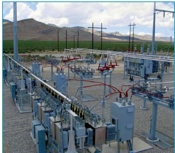
AMSC Transmission SVC Deployment in Western United States.
